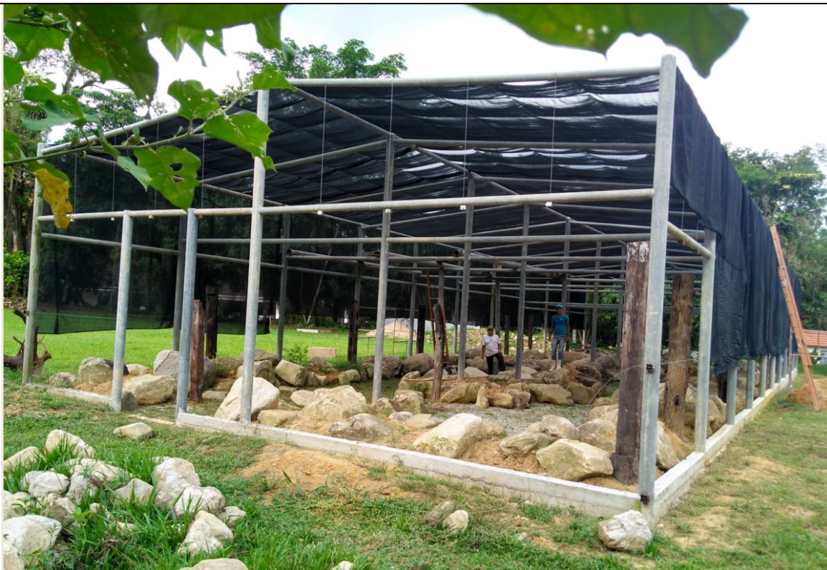
Fig 5. The 70% sun filter mesh took a long time to sew together. June 2019
