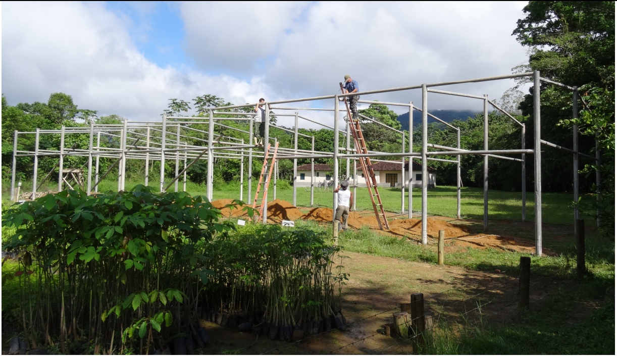
Fig 3. The tubular construction provided a sturdy structure in March 2019
