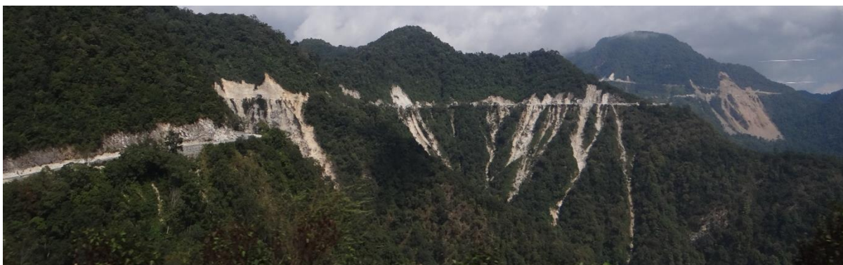
Figure 6. Road construction through rugged terrain and orchid habitat
